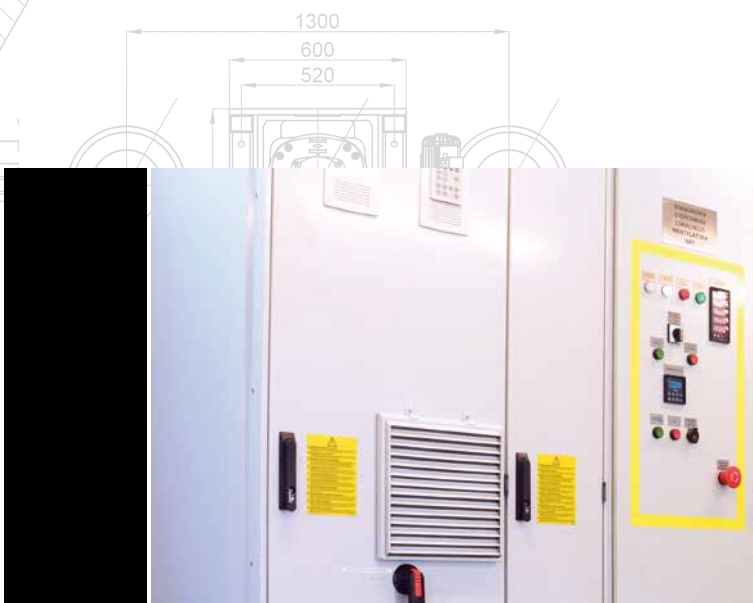
phot. 7 RW 400/230 V auxiliary switchgear
